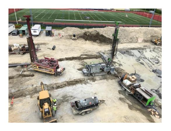
Photo 1 – Completion of Lateral Geothermal Piping Installation in field #1.
